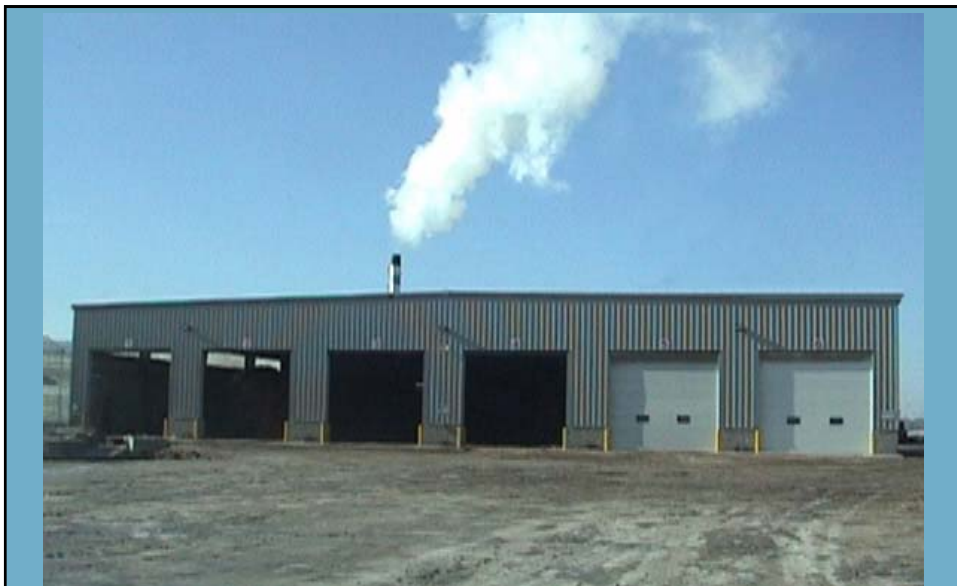
A new wood storage building (in Kingsville, Ontario) 80 MMBTU/hr
