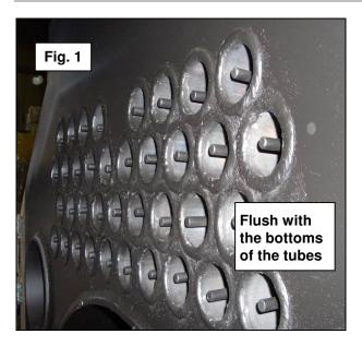
Remove the displacement rods with a pair of pliers, as shown below. The heat exchanger should be cleaned at the intervals prescribed so that, on the one hand, performance and efficiency are maintained, and on the other, the displacement rods can be easily removed.
