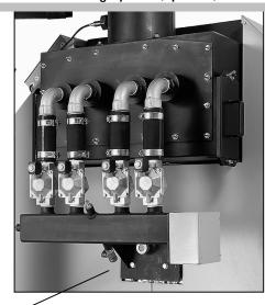
Regularly drain condensation water in the compressed air distribution bar.
