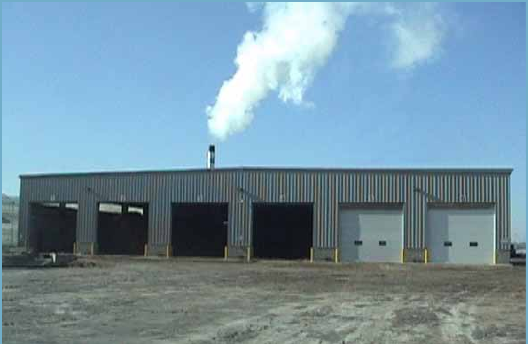
A typical wood storage building (in Kingsville, Ontario)
