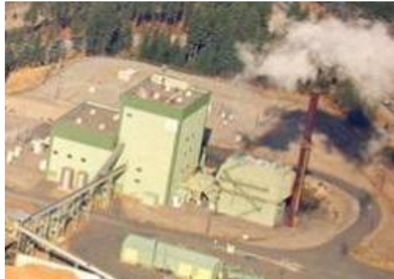
30 MW ABB/Zurn biomass plant, CA
