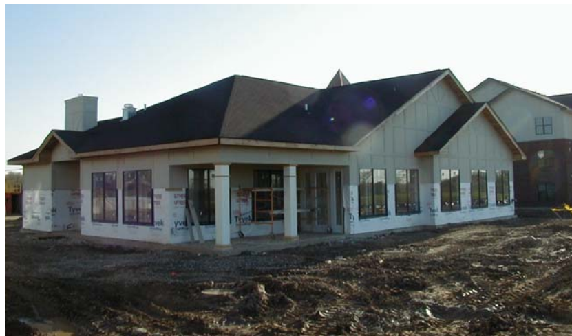
Southwest view of the Community Building during construction
