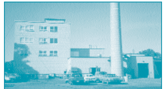
A Stack at the Prince Edward Home (Seniors Facility) Charlottetown, PEI District Heating, 1985
