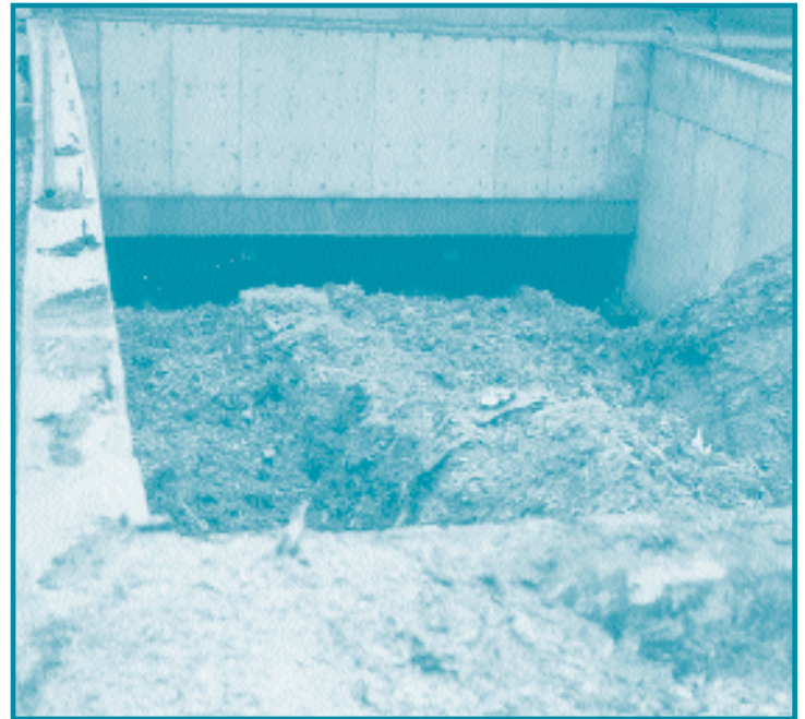
In-ground Concrete Storage Bin
